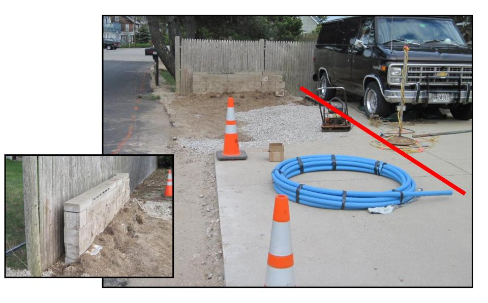
A buried course of old stone remains in the right of way. It is expected that this will be removed and replaced with "slip form" curb for consistency with the rest of the design on the other side of the road and other side of the motel office driveway.
