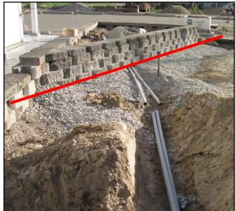
The pavement was cut precisely on the property line along the motel's parking (Depot St.). The Cement Drive installed on the right of way should be cut back to the property line also, or perhaps even a bit more to provide the owners with the ability to bury underground electrical conduit on their property after it is removed from the right of way.
